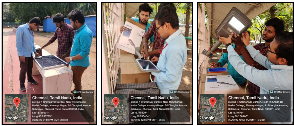
Installation of Solar Light
